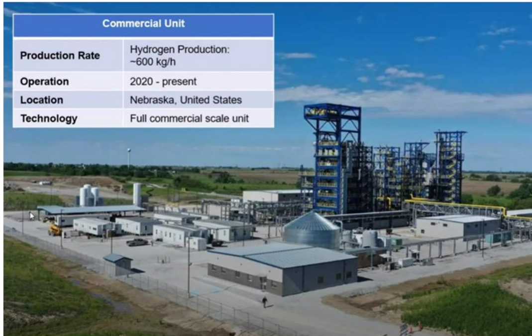
Monolith Corp. – Olive Creek Plant phase 1 Hallam, Nebraska
